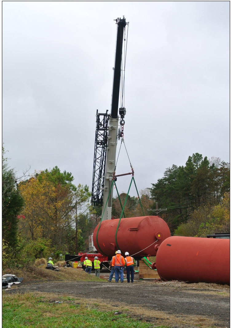
Abandoned tanks at the Y-12 Complex
