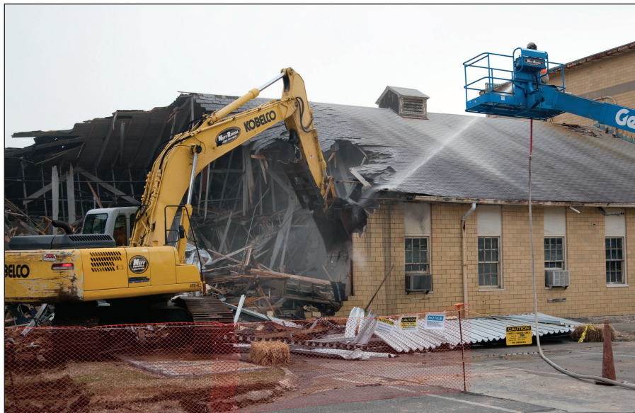
Building 9735 has been demolished
