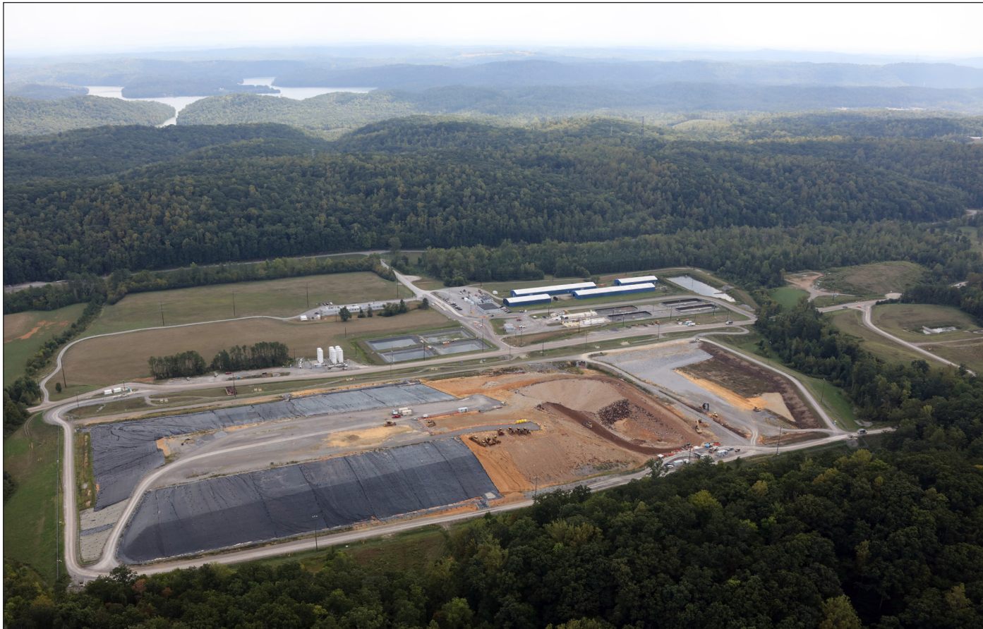
Environmental Management Waste Management Facility
